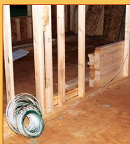
147 | Pulling Cable in New Construction
