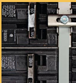
319 | From Generator to Switch
