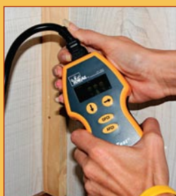
203 | Troubleshooting an AFCI Circuit
