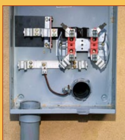
78 | Connecting Meter Base to Panel
