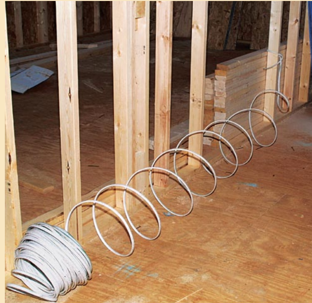
Letting the cable spin out will leave it in spirals—making it impossible to pull it through the studs.
