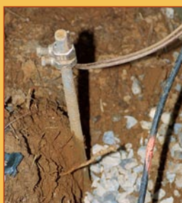
118 | A Low- Resistance Panel-to-Earth Ground
